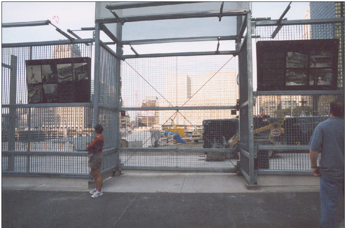
View of the public viewing area (facing north) and information boards at the WTC Site 8
